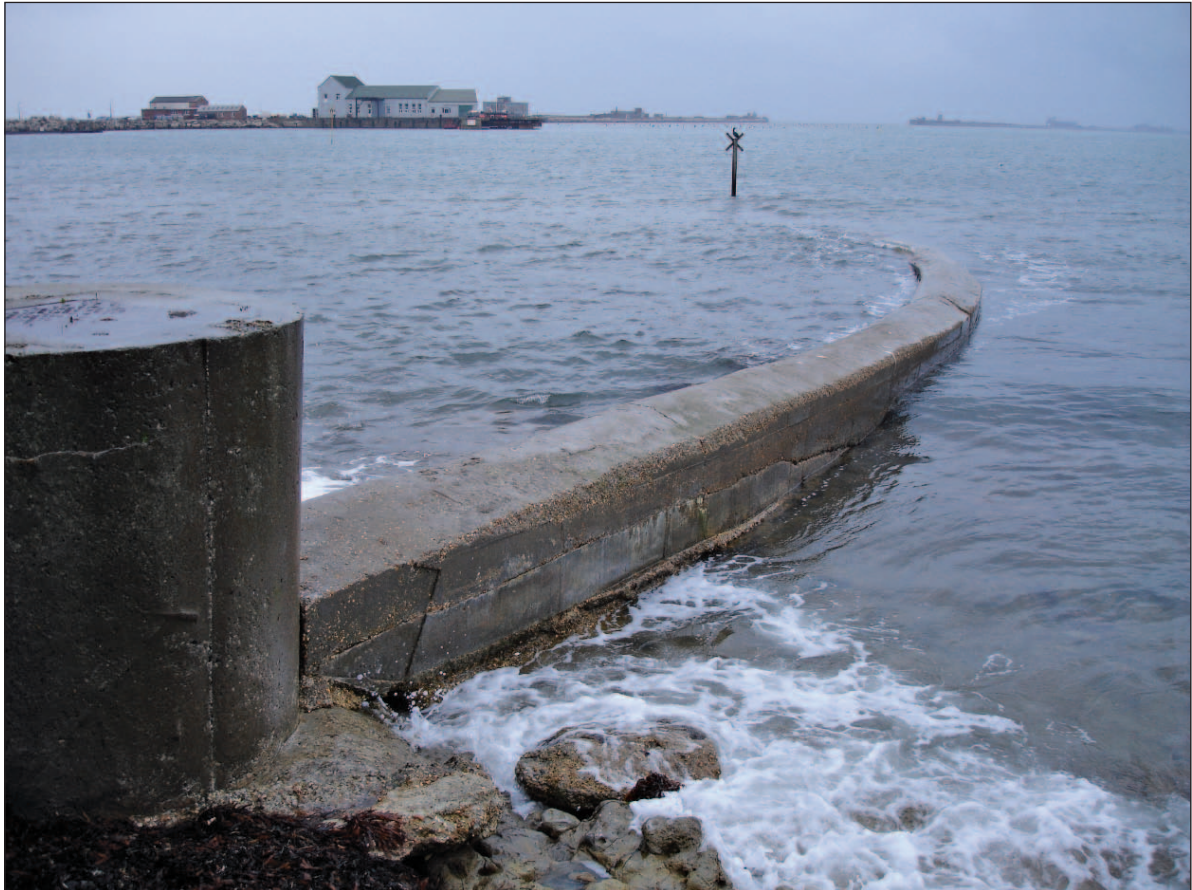
Figure 8.1: A pipeline discharge.
