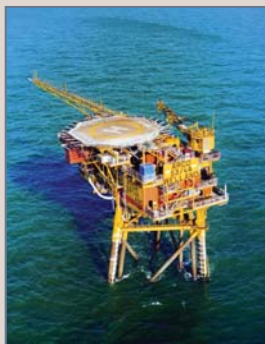
Welland gas platform in the southern North Sea
