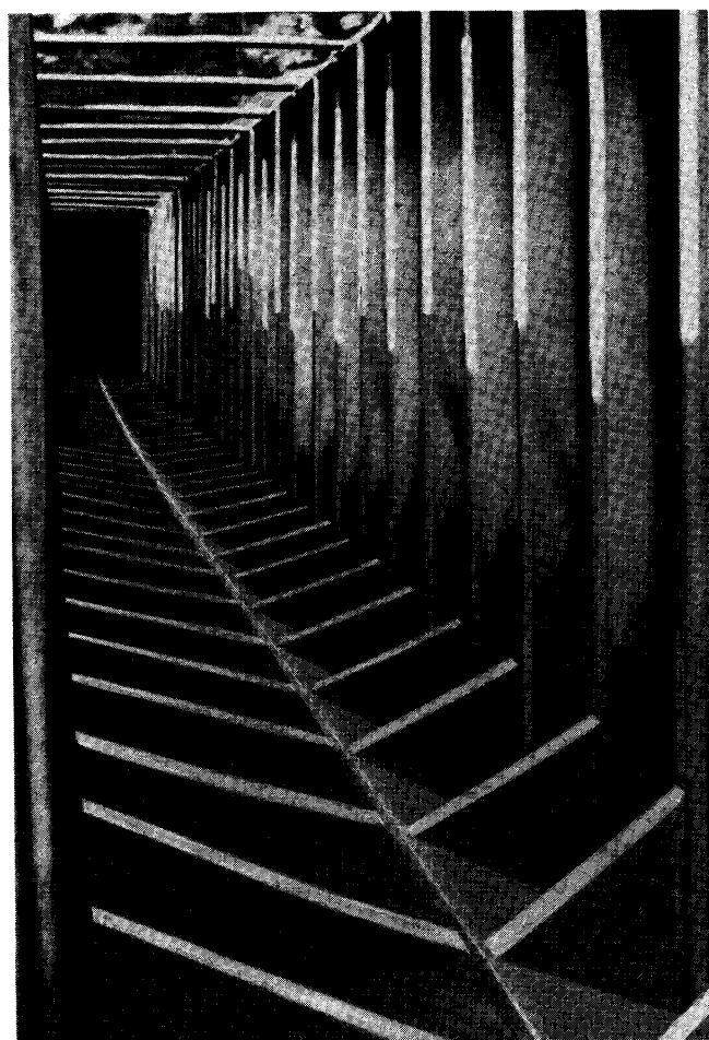
Figure 26 A view through the prefabricated Alaskan 'Model A' Denil fish pass.
