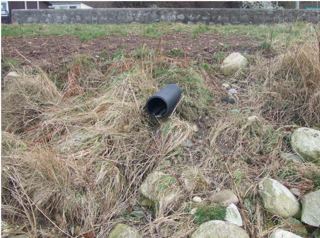
Figure 36. Black pipe under road, no flow
