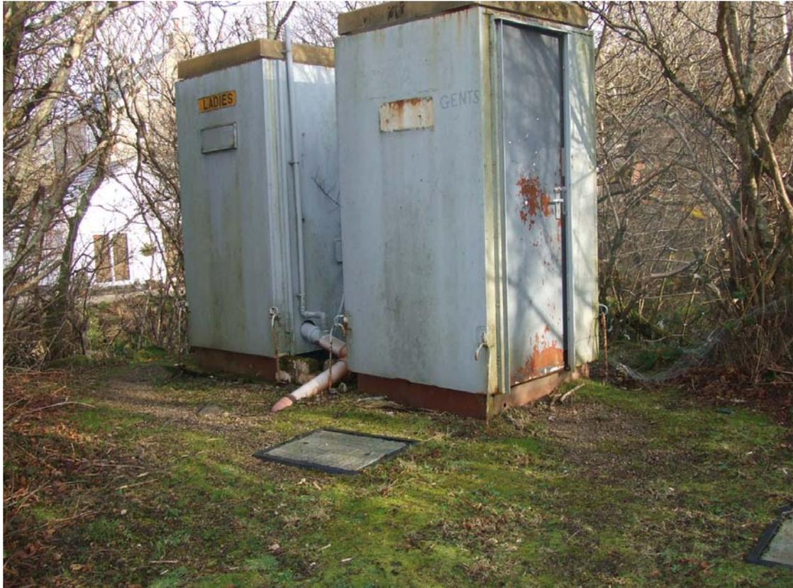
Figure 30. Pirnmill public toilets with inspection covers and suspected septic tank
