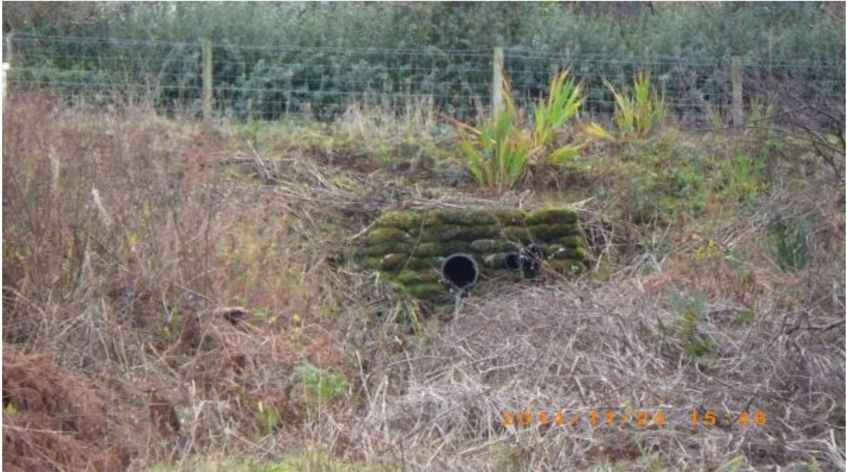
Figure 13. Watercourse diverted under road via pipe associated with wp 33.
