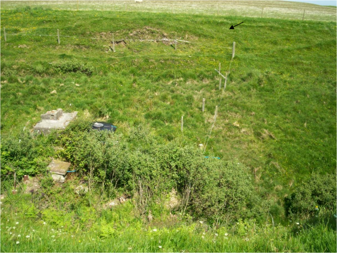
Figure 9. Septic tank on west shore
