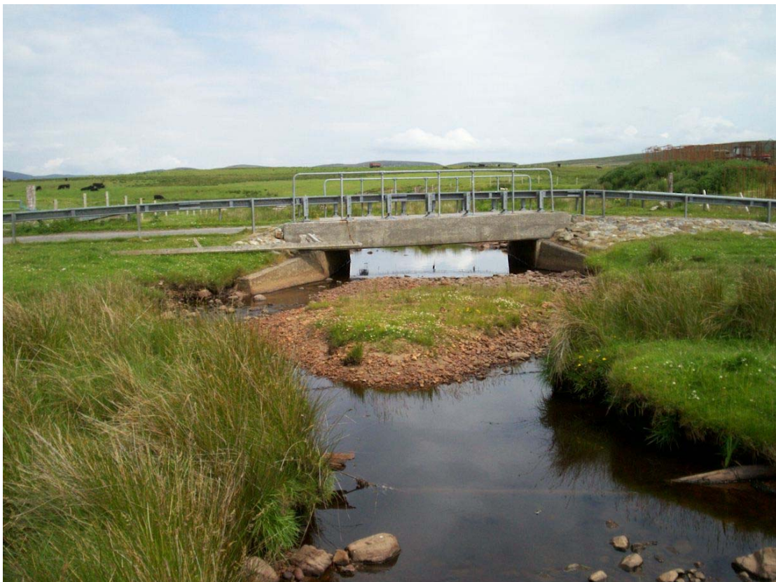
Figure 16. Stream at southern end of trestles
