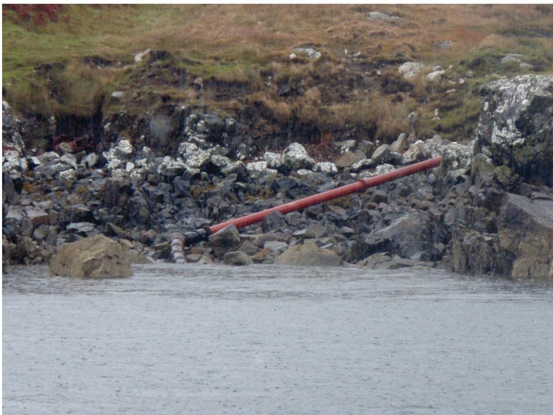
Figure 8. Sewage discharge pipe for Loch Leurbost in Outer Loch Erisort
