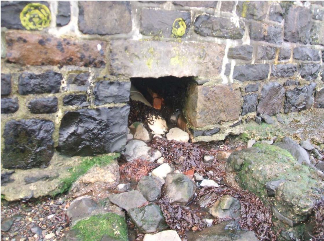
Figure 11. Probable septic tank outlet
