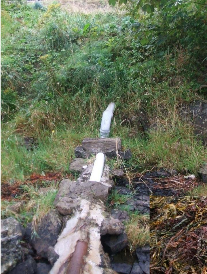
Figure 16. Probable septic tank outlet
