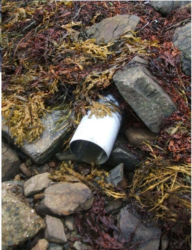
Figure 17. Probable septic tank outlet
