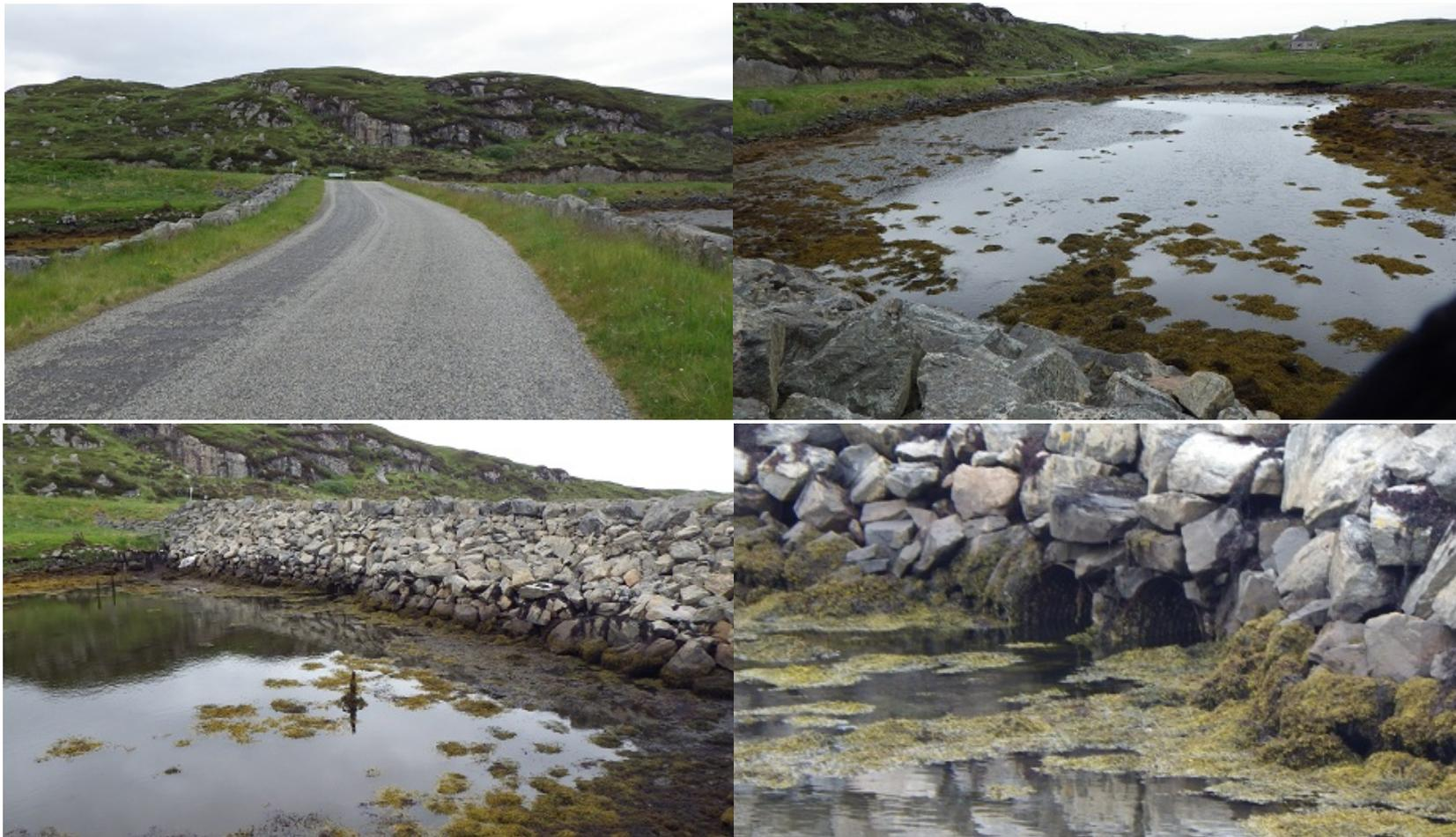
Figure 16. Road causeway across loch inlet with corrugated pipes allowing flow under road. Waypoint 29.
