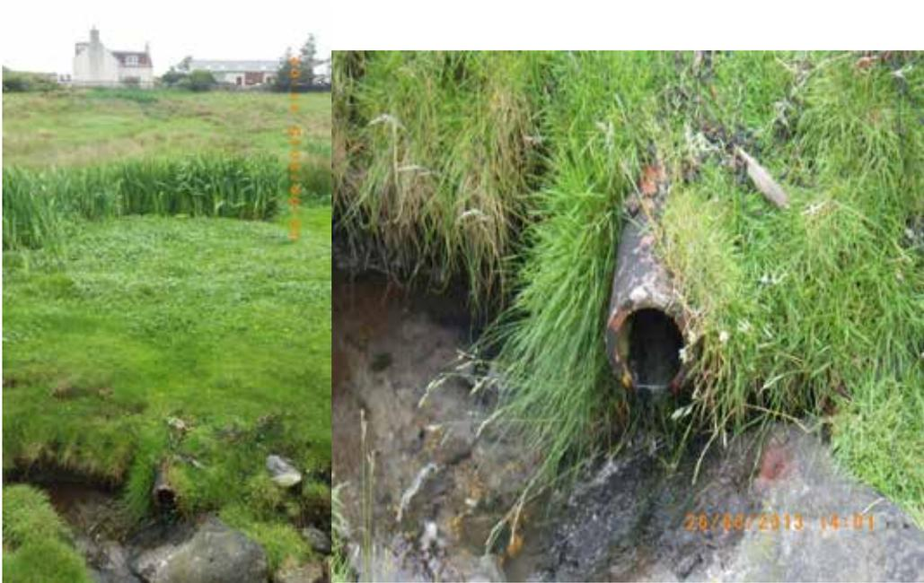
Figure 18. Pipe discharging into watercourse from below house. Waypoint 38.
