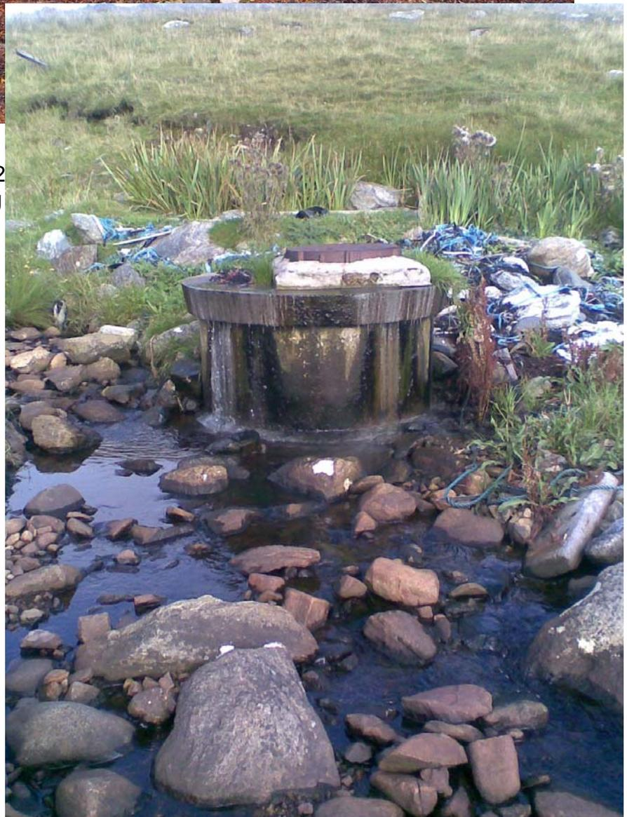
Figure 35. Roag080765 Septic discharge with human waste on shoreline, N of Circebost.
