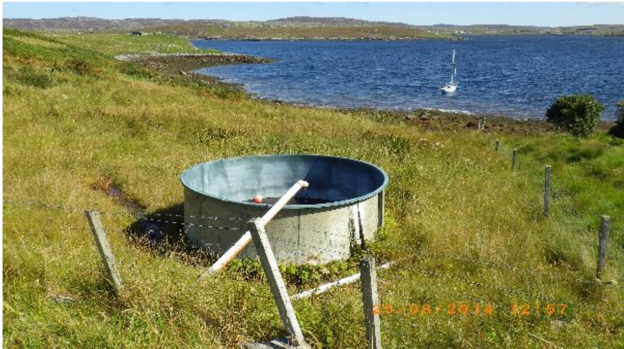
**Fig 11:** Large, open tank below public road, with pipe and inflow running in. Waypoint 45.
