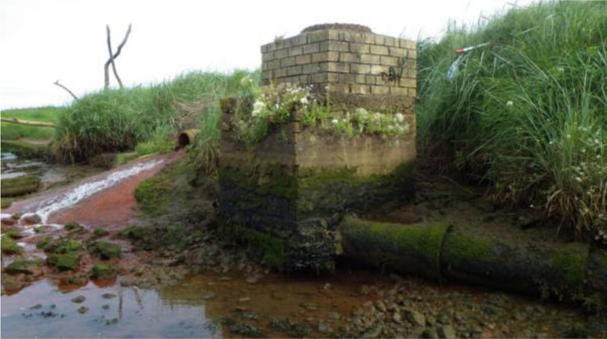
Figure 17 Inspection junction in pipe (leaking) connecting with St. Andrews Caravan Park PS EO. Location of unplanned freshwater sample MCFW8, Waypoint 39.
