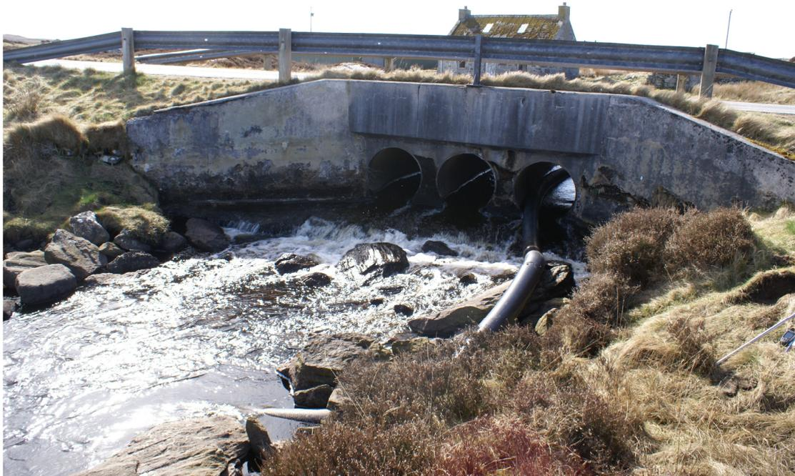
Figure 4. Pipes under road, each approx. 1 m wide
