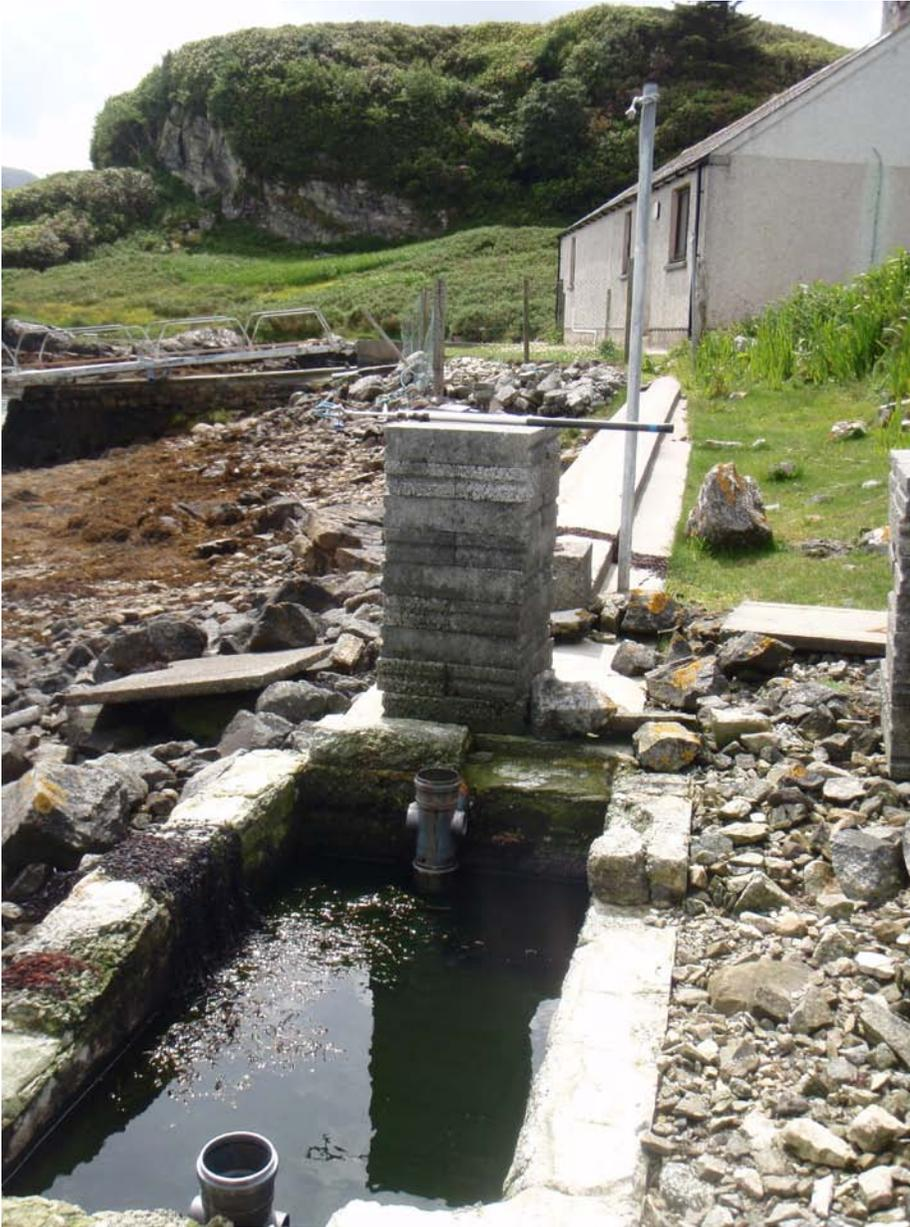
Figure 12. Open septic tank leading from workshop
