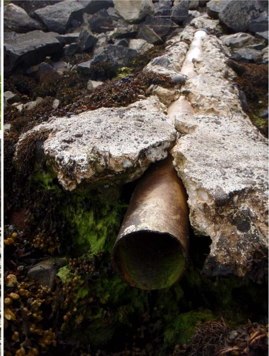
Figure 13. Dry outfall pipe leading from workshop septic tank
