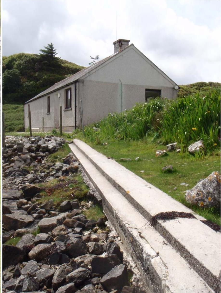
Figure 11. Outfall pipe covered in concrete leading from workshop
