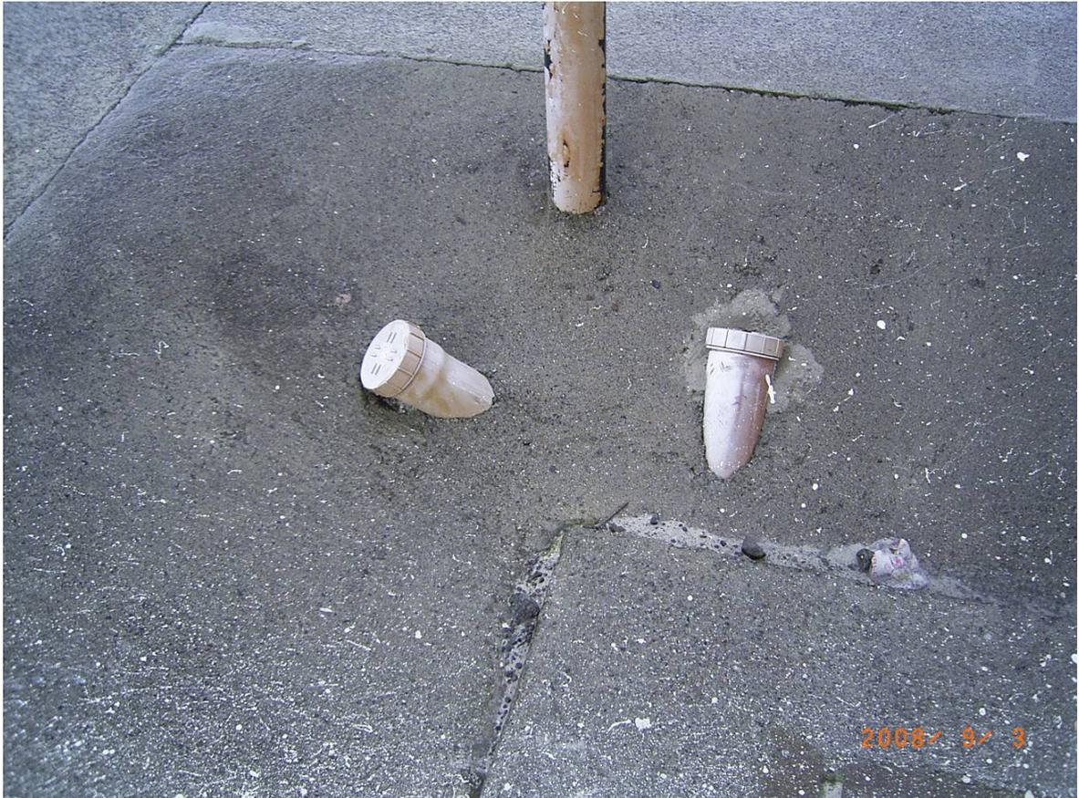
Figure 4 Presumed air terminal septic tank vents
