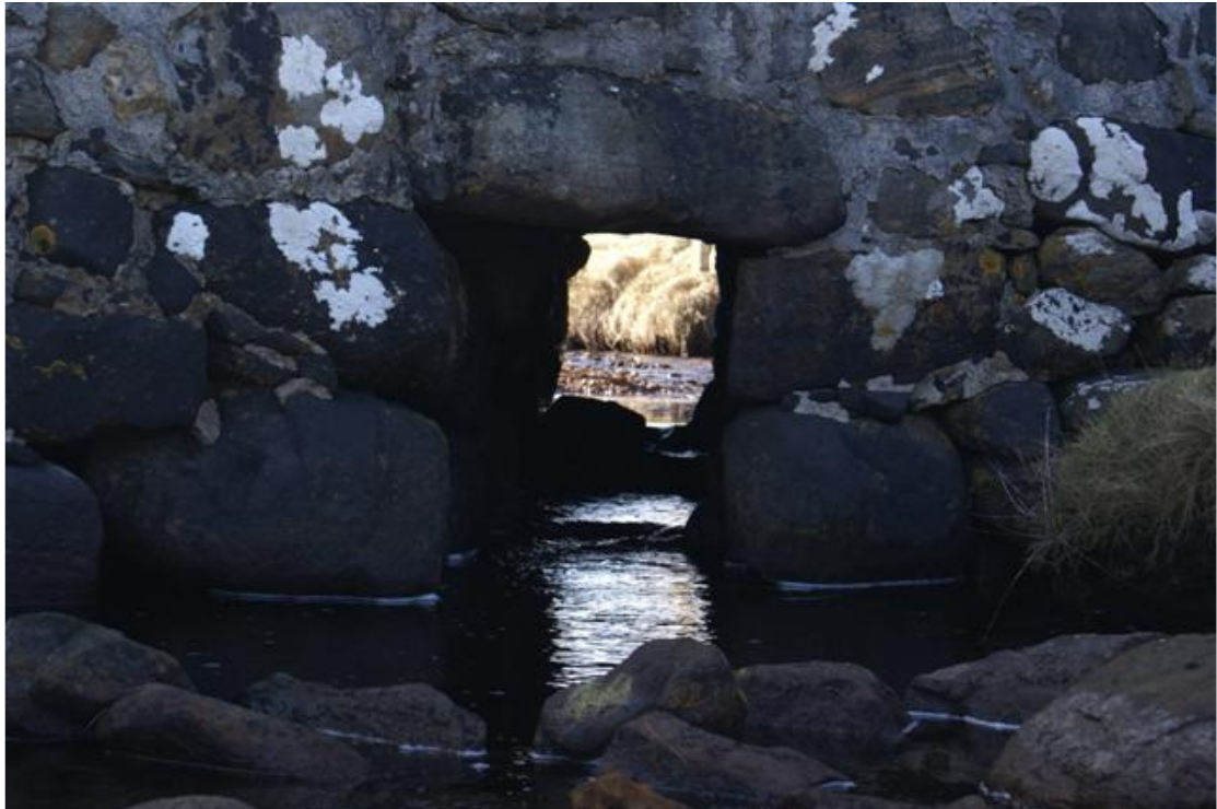
Figure 4. Culvert flowing under road
