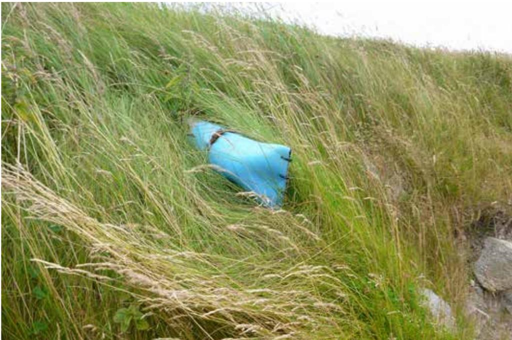
**Figure 7 – Capped pipe associated with the septic tank in Figure 6.**
