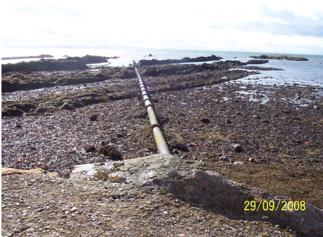
Figure 30. Pipeline believed to be overflow for a mid line pumping station that pumps sewage to the pumping station at Anstruther or St Monans
