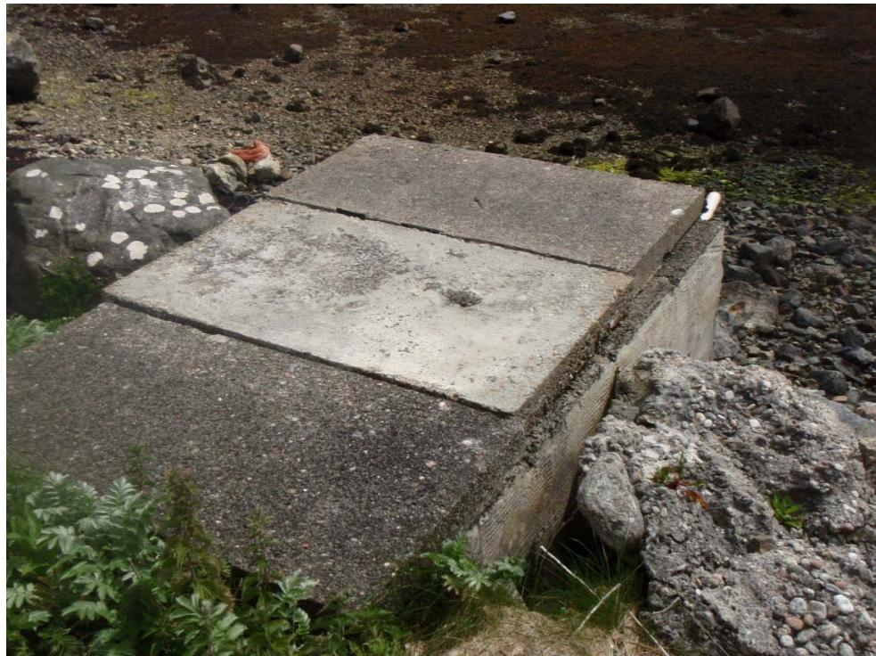
Figure 14. Outfall pipe covered in concrete slabs
