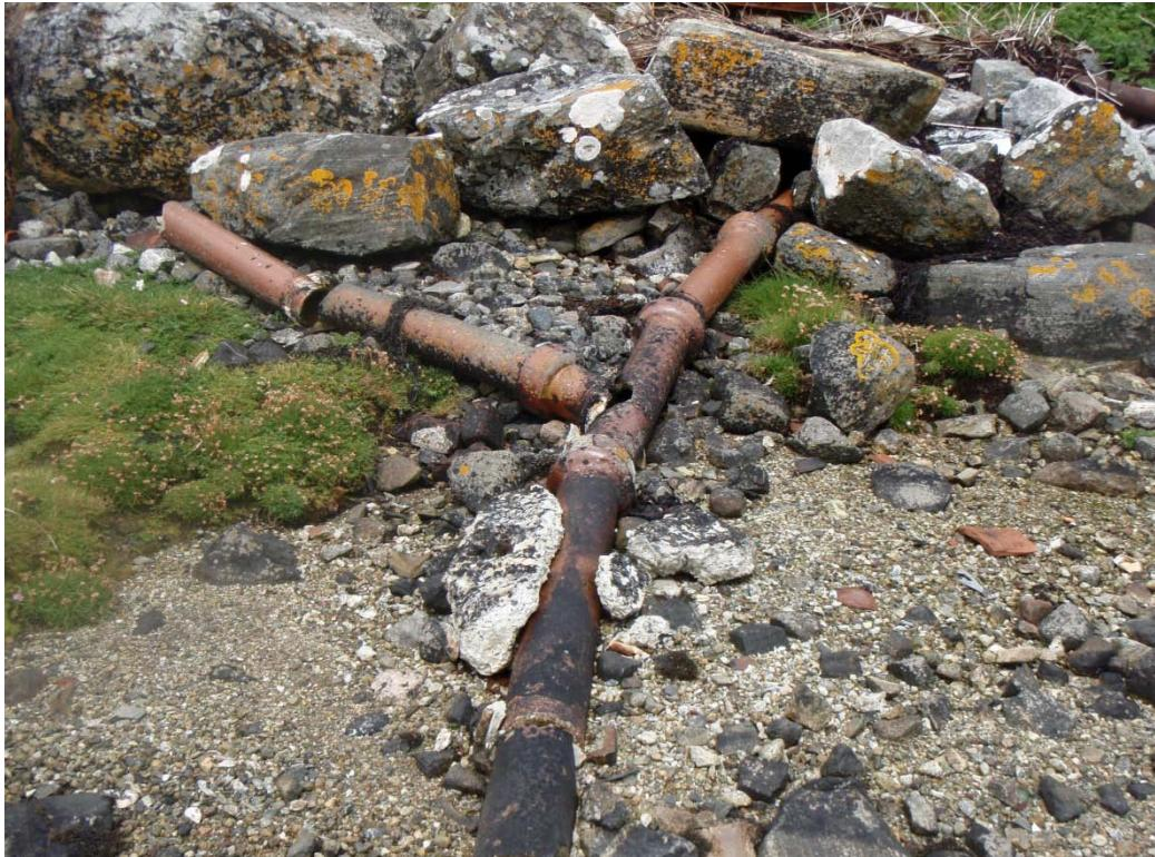
Figure 16. Broken pipe, no flow
