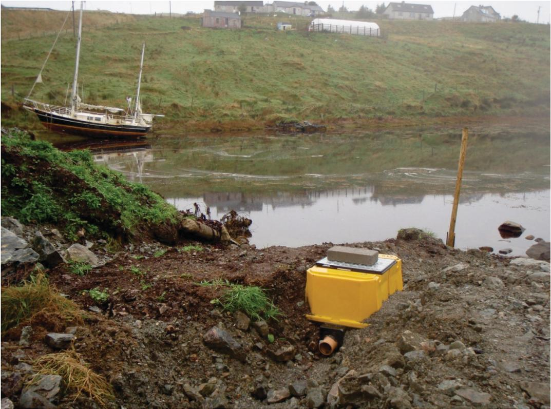
Figure 12. New septic tank at Tòb Garyvard
