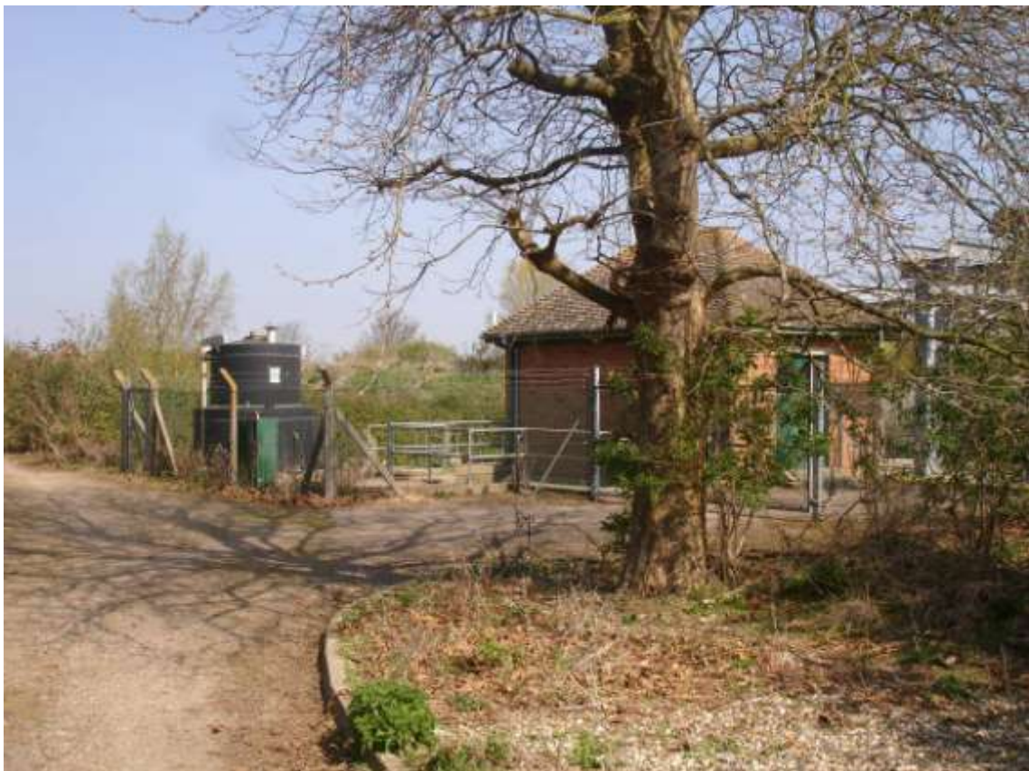
Figure XIII.7 Main Maltings Pumping Station entrance.
