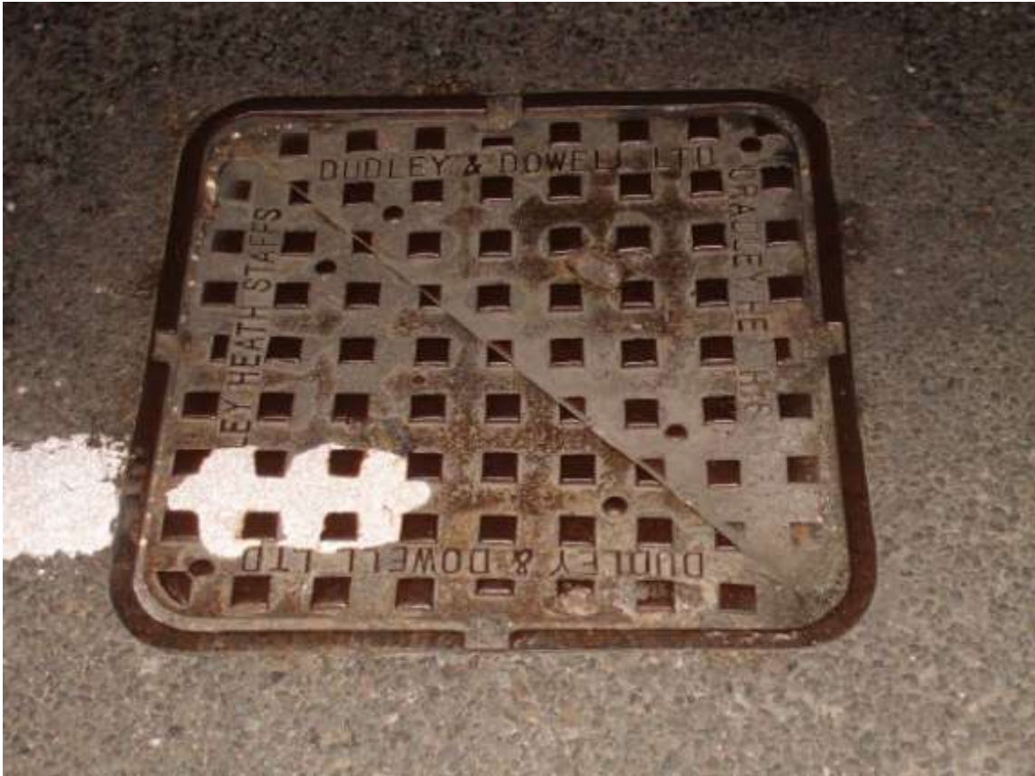
Figure XIII.5 Manhole cover at Hervilly Way and Walton Road Overflow.
