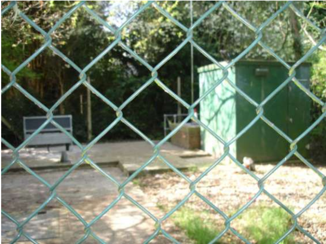
Figure XIII.6 Kirby-le-Soken Pumping Station entrance.
