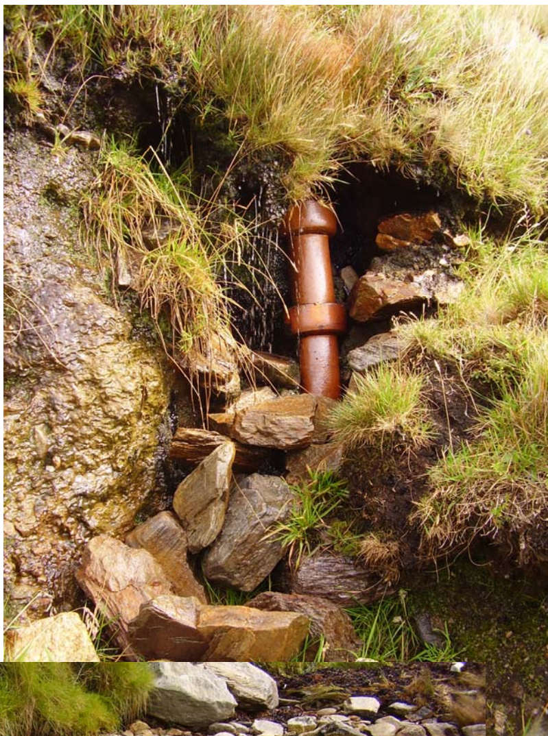
Figure 24. Vertical section of pipe discharging onto shoreline
