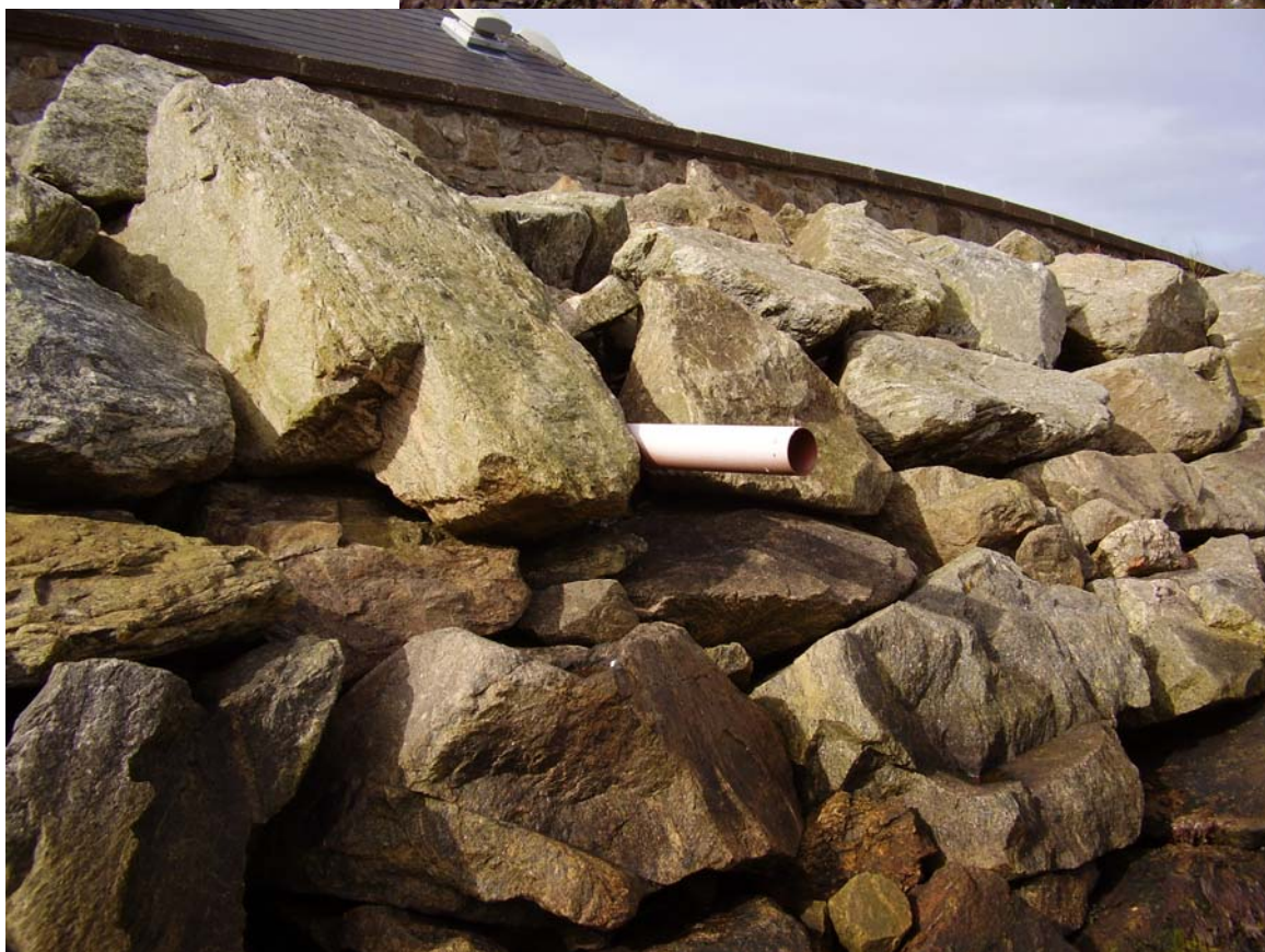
Figure 11. Drain pipe through seawall.
