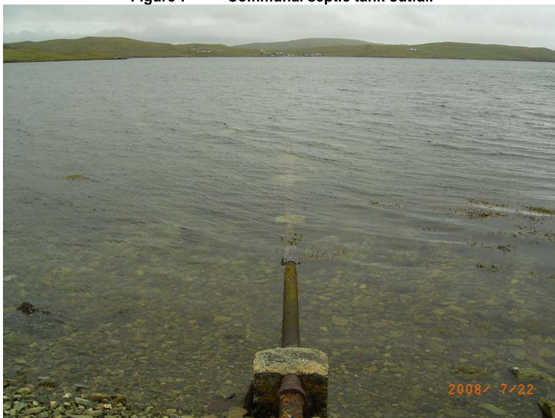
Figure 7 Communal septic tank outfall
