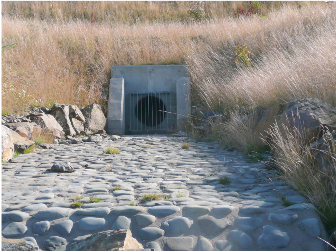
Figure 12. New culvert
