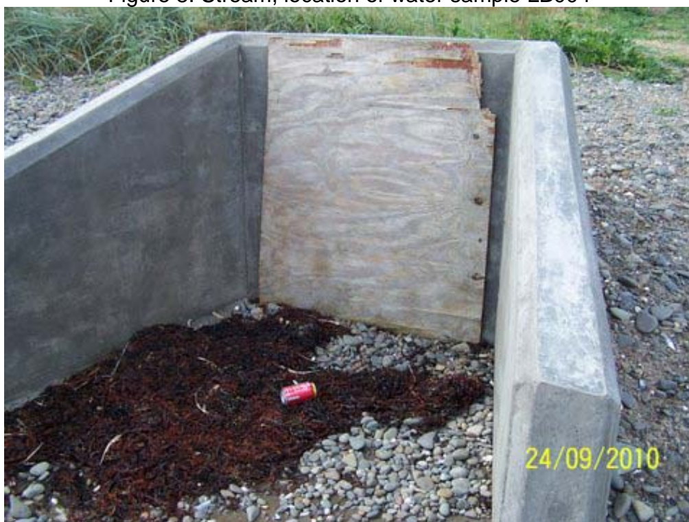
Figure 9. New culvert – boarded up
