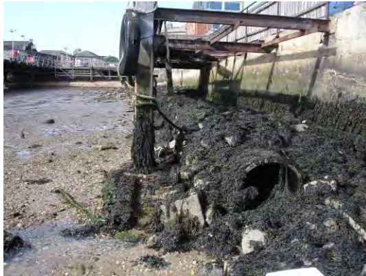
7: Pipe at Hythe slipway
