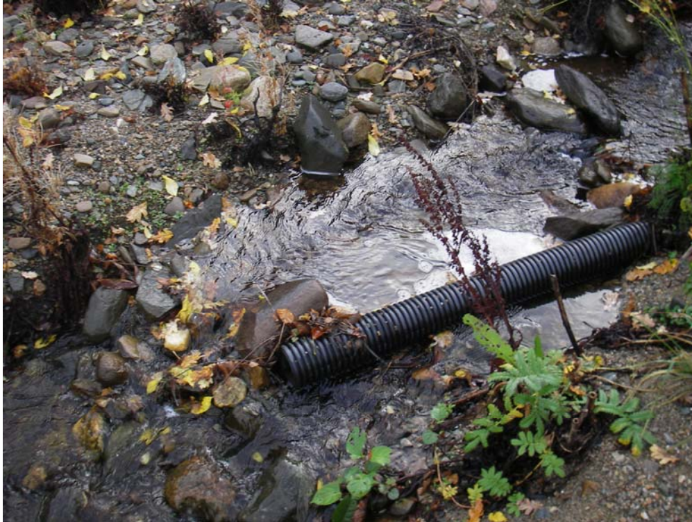
Figure 13. Presumed septic tank outlet
