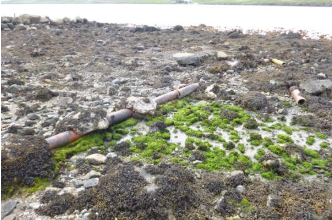
Figure 11 – Broken pipe with a grey discharge associated with a septic tank below a house in Brae.
