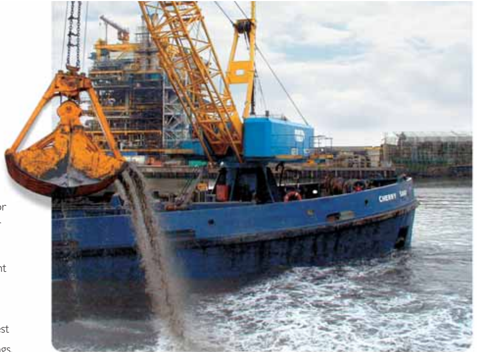
Harbour maintenance dredging, Lowestoft
