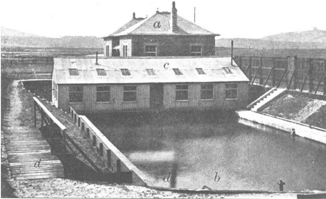
Plate 4. Part of the former Marine Laboratory and hatchery site at the Bay of Nigg, Aberdeen, showing the Laboratory (a), and the tank house (c) partly built over one end of the spawning pond. The pond had a capacity of 160,000 gallons (728,000 litres) and could be filled or emptied, via a pipe at (d), according to the state of the tide. The tank house was erected in 1901-02, funded by a £200 grant from Aberdeenshire County Council. In return the Board agreed to give technical instruction to fishermen at the Laboratory for a period of 5 years.
