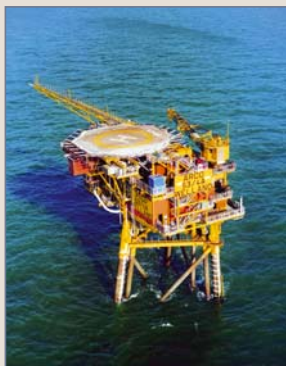
Wellgas gas platform in the southern North Sea
