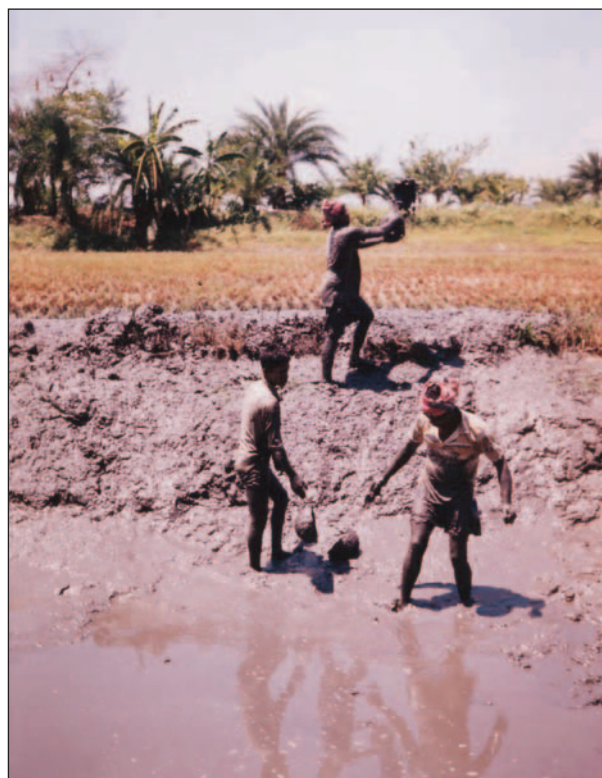
Gher construction by labourers
